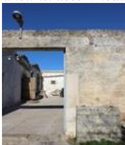
Figure 4. View of Masseria Losurdo Farmhouse.
